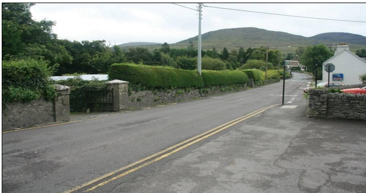
Plate C2: Access point from the Pier road is particularly dangerous at present. The County Council should be approached and asked to install speed ramps at this location. In addition no signage exists to indicate entrance to the park at this location. It is recommended that signage and access be improved.
